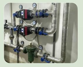
The heat network has been replaced with preinsulated pipes
